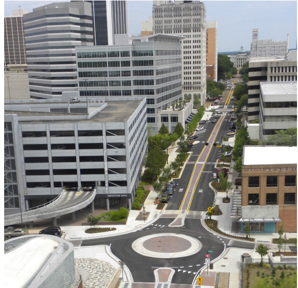
Aerial view of reconstructed Capitol Street in downtown Jackson, Miss.
